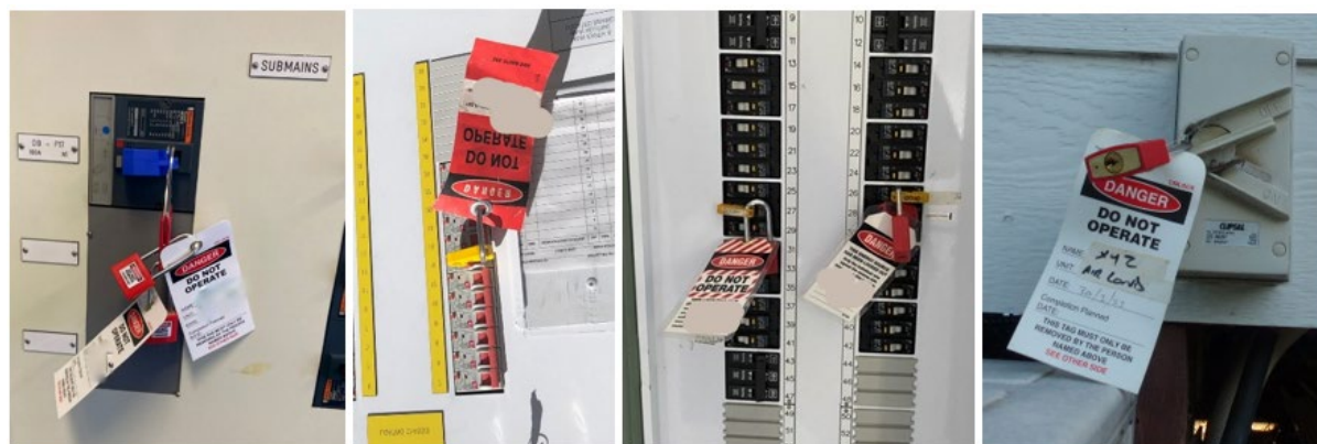
Figure 1 – Examples of locking methods incorporating danger tags.
