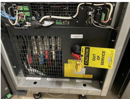
Figure 4 – Examples of locking methods incorporating out of service tags.
